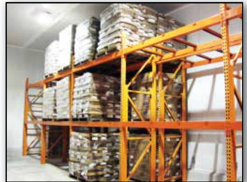
Double deep pallet rack is an economical space maximizer.
